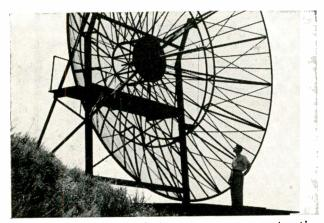
**This giant transmitting antenna** creates the beam for experimental antenna pattern measurements – part of the Hughes microwave research and development programs.
