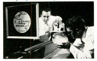
Engineers at the IBM Federal Systems Div. Laboratory check out part of a new air navigation system under development. System uses a computer to automatically position a map of half the earth inside a glass hemisphere in such a way that the area over which the plane is flying is projected on a display screen.
