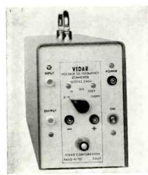
can be switched from 0.1 v. through 1000 v. in 5 steps. Input polarity is indicated automatically. Applications include: Analog-to-digital conversion (used with a counter), precise integration, and telemetry. Three package designs are available. Model 240A. Vidar Corp., 2107 El Camino Real, Palo Alto, Calif.
